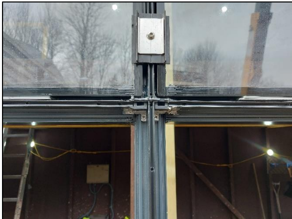
Photograph No. 14 - Cruciform joint details
