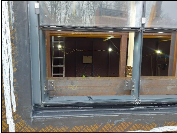
Photograph No. 17 - Bottom LHS with glazing removed
