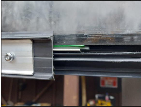
Photograph No. 12 - Glazing packers
