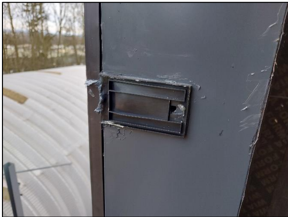
Photograph No. 10 - Transom connection on mullion
