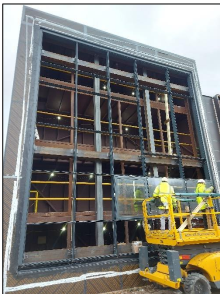
Photograph No. 8 - Full sample with glazing removed
